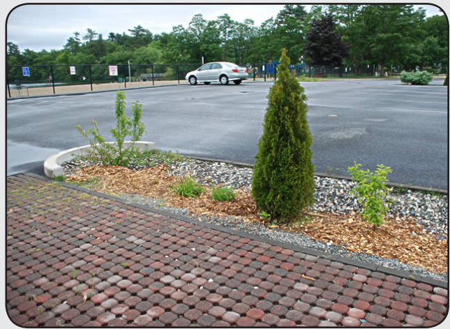
LID includes design elements like porous pavers and rain gardens that let water soak into the ground.
