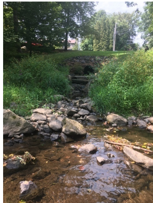
Figure 2-15: Examples of stormwater outfalls that discharge to impaired segments of the Pomperaug River in Southbury, CT. (Photos by Fuss & O’Neill, Inc.)
