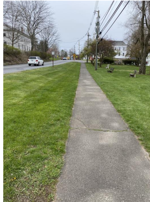
Image 2 (Above): Proposed location of vegetated swale between Main Street and existing sidewalk. Curb cuts would allow stormwater to enter the swale from the roadway.
