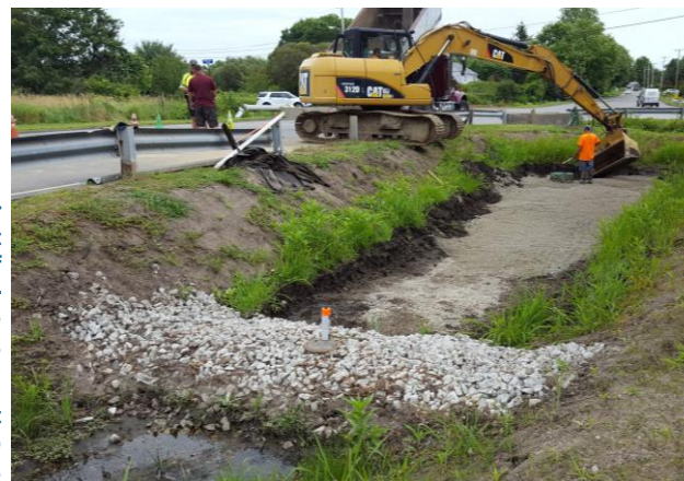
Above: Existing conditions on Rte. 6 just north of Scratchville Road (looking South). Sediment and debris accumulation indicates ponding and bypassing of existing catch basin during high-intensity precipitation events.
