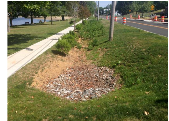
Image 3 and 4 (Above, Left): Examples of vegetated swale receiving roadway runoff via curb cuts.
