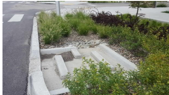
Image 1: Example of an established bioretention basin with a concrete curb cut and concrete pretreatment structure to remove sediment before runoff enters the planted portion of the basin.
