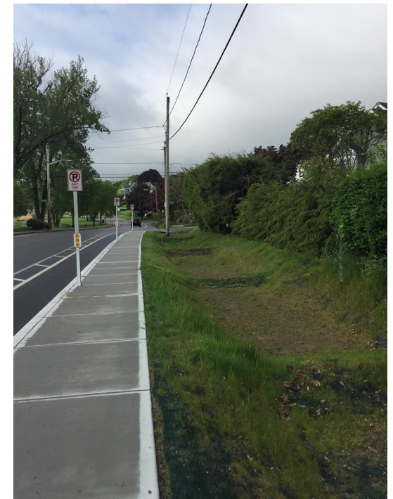
Image 3 (Right): Example of swale with check dams to slow and infiltrate water.
