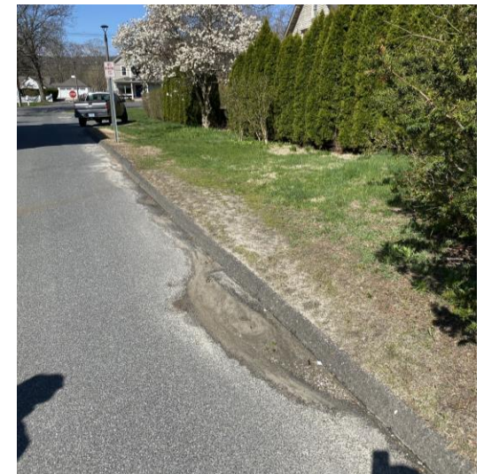
Image 2: Significant sediment accumulation at an existing catch basin at the upper end of the site indicates a potential erosion problem on the upgradient hillside.
