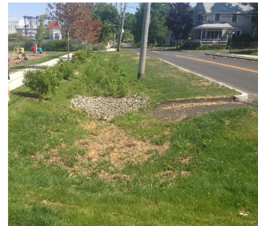
Image 2 (Above): Proposed location of vegetated swale between Main Street and existing sidewalk. Curb cuts would allow stormwater to enter the swale from the roadway.
