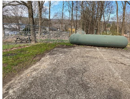
Image 1: Existing 1,000 gallon aboveground storage tank and proposed area for bioretention at the upper parking lot. Field observations indicate that stormwater runoff currently ponds in this corner of the parking lot.
