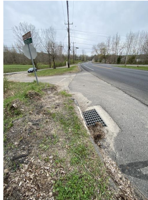
Above: Existing conditions on Rte. 6 just north of Scratchville Road (looking South). Sediment and debris accumulation indicates ponding and bypassing of existing catch basin during high-intensity precipitation events.
