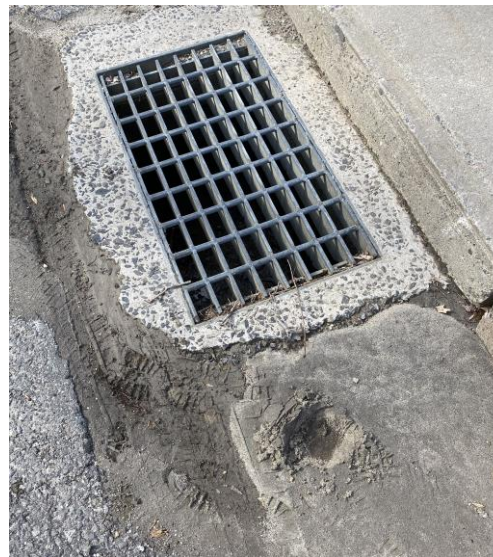
Image 2: Significant sediment accumulation at an existing catch basin at the upper end of the site indicates a potential erosion problem on the upgradient hillside.
