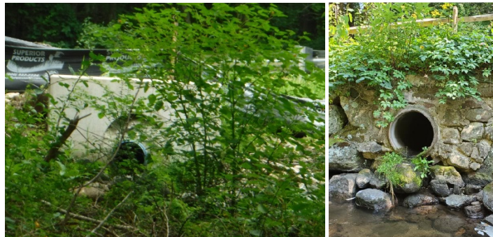
Figure 7. Examples of stormwater outfalls that discharge water in catch basins located on roadways and other impervious surfaces; their associated network of drainage pipes discharge stormwater away from the roadway and onto the ground or into a nearby river /stream.
